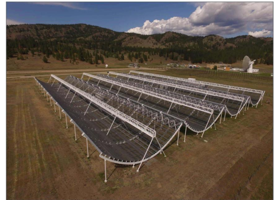
Transit telescope = a large field-of-view and a high discovery rate
